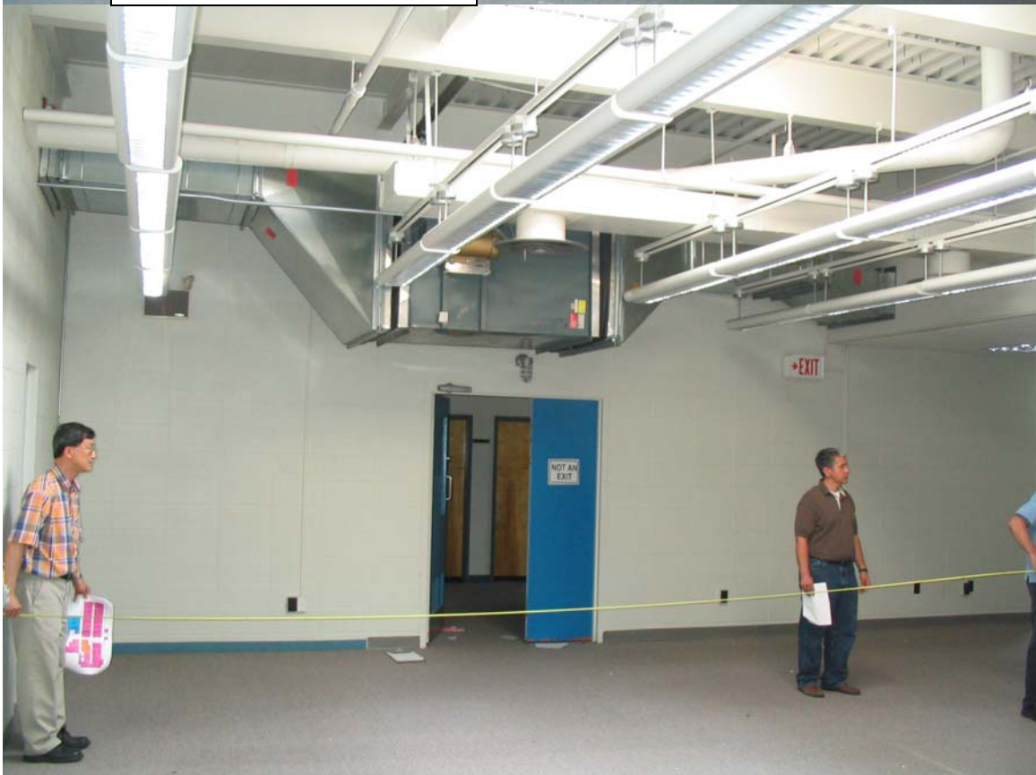
Nice bright room at east end of second floor. All internal walls can be removed. Pillars leave enough space.
